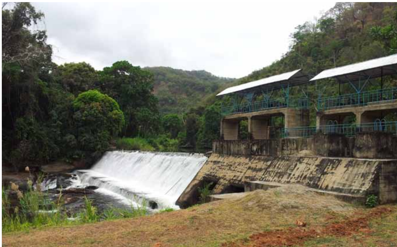
KPL hydropower reservoir and weir, Mngeta River.
