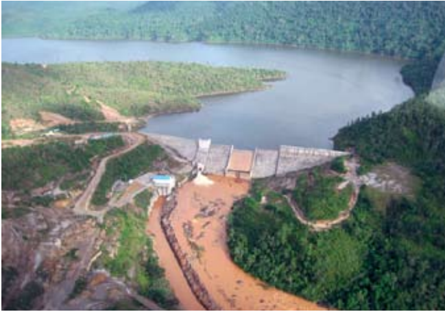
The Chalillo Dam in Belize is one of many large dams with major problems with sedimentation. Photo: Probe International
